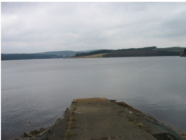
Remnants of the old railway line, now running straight into the lake
